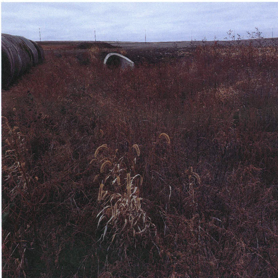
Figure 6. Overview of disturbance from culvert and excavated ditch, facing west-northwest.
